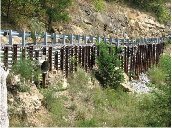
Road construction on slopes underlain by shale often requires additional foundation support to prevent pavement failure. Proper drainage maintenance is also essential. Photo by Dan Carey, Kentucky Geological Survey.
